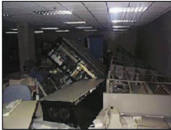
LEFT: Computers in a server room were not seismically restrained before the Feb. 28, 2001 Nisqually, Wash. earthquake.
